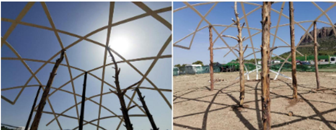
Figure 17: Own Spirit 2019 Gridshell, final construction.
