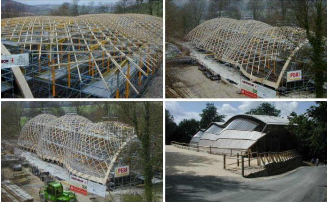
Figure 4: Weald and Downland gridshell erection process [10]
