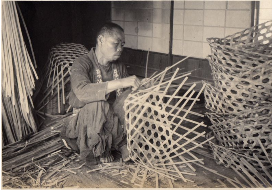
Figure 01: Image of Japanese basket maker working with the kagome lattice
