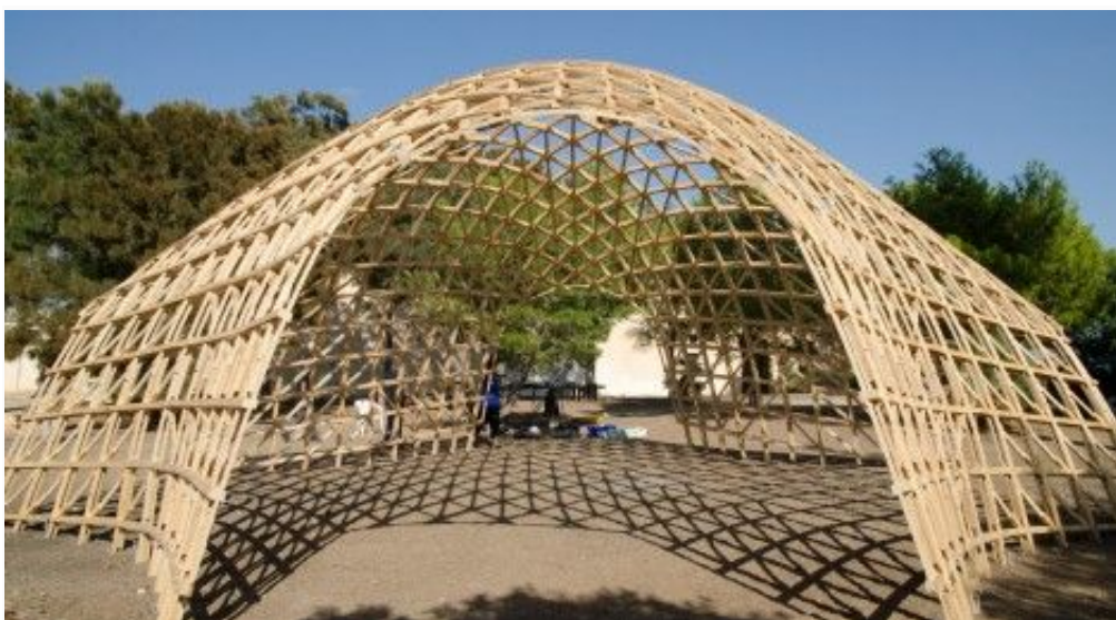
Figure 12 : Image of the Toledo Gridshell structure built
