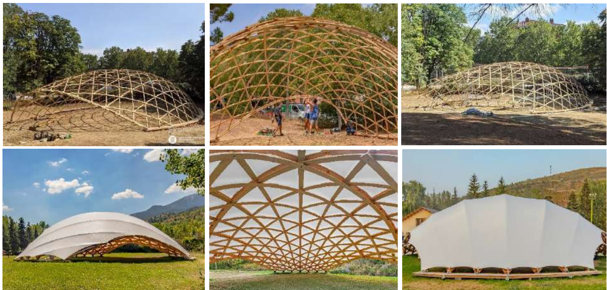
Figure 7. a) Top three images; Chebyshev grid shell made of 1 layer, plywood 5x2cm. Location: Escuela Técnica Superior de Arquitectura del Vallés (ETSAV). b) Bottom three images; 3 ways Geodesic grid shell made of 2 layers, plywood 13x1.5 cm. Location: Alp, Catalonia, Girona
