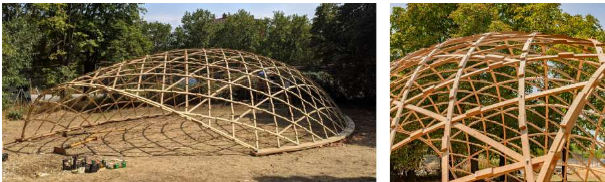
Figure 4: Gridshell built at the campus of the Escuela Técnica Superior de Arquitectura del Vallés (ETSAV).
