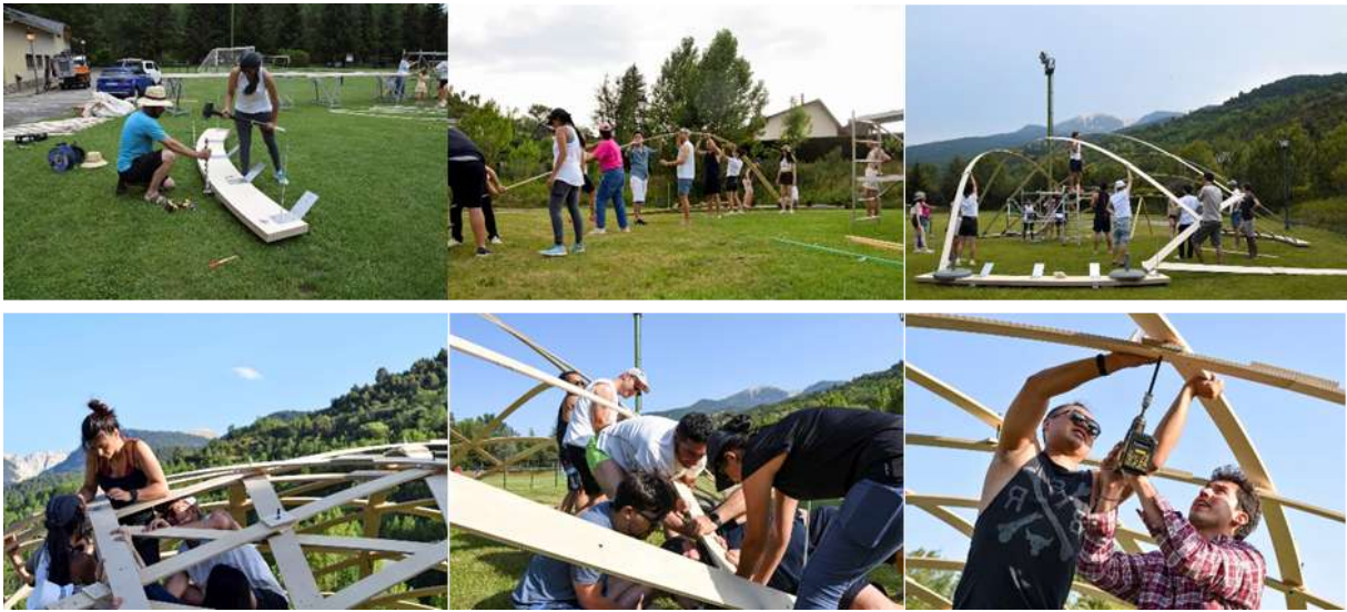
Figures. Construction process.
