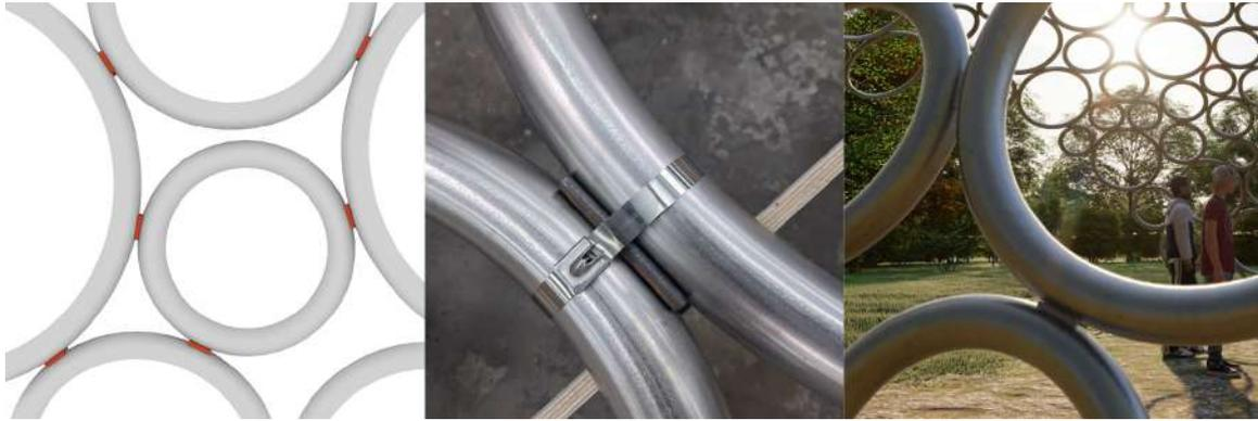
Figure 21: Steel rods for reinforcing and bridging welded joints
