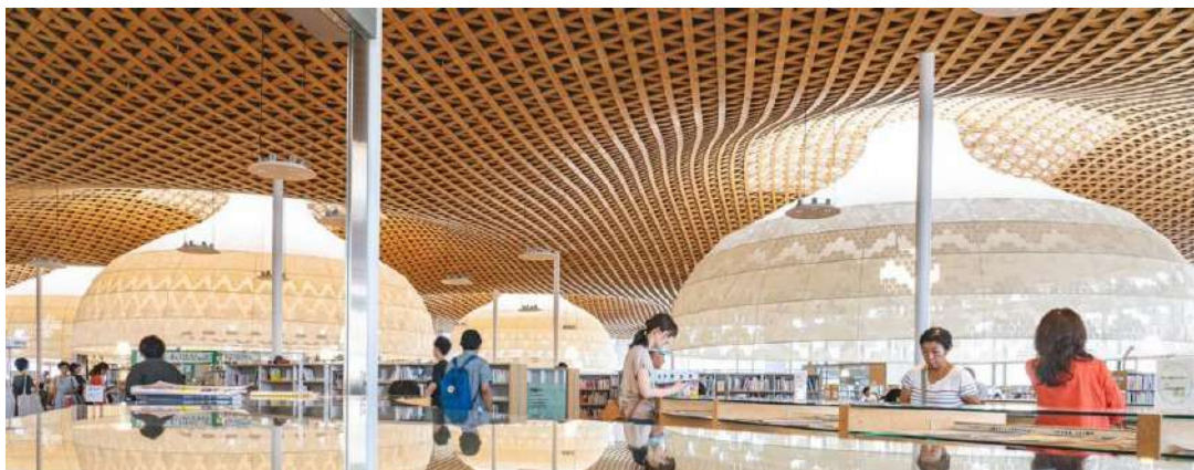
Figure 1. Toyo Ito's "Minna No Mori" Gifu Media Cosmos' triangular lattice roof.
