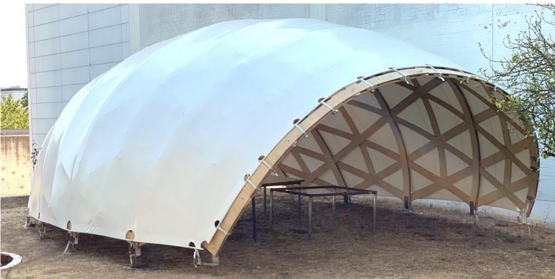
Figure 19. a) Initial three arches from first curve family being erected. b) First three arches from family one with locking arches from families two and three in place. c) Completed timber structure. d) Pavilion with membrane tightened and in place.
