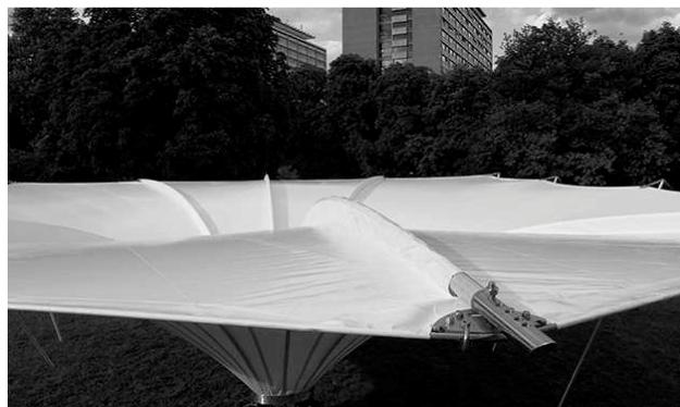
Figure 33: Special device for tangential prestress. [10]
