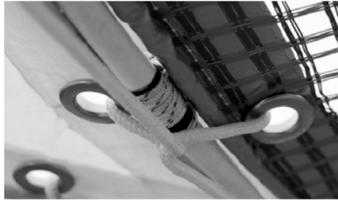
Figure 34: Special device for tangential prestress. [10]
