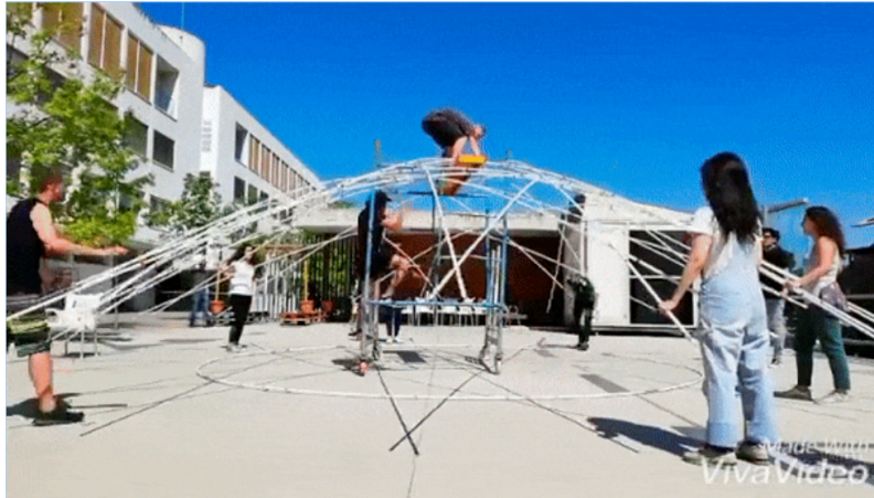
Figure 102: Structure up the scaffold being joined with swivel couplers
