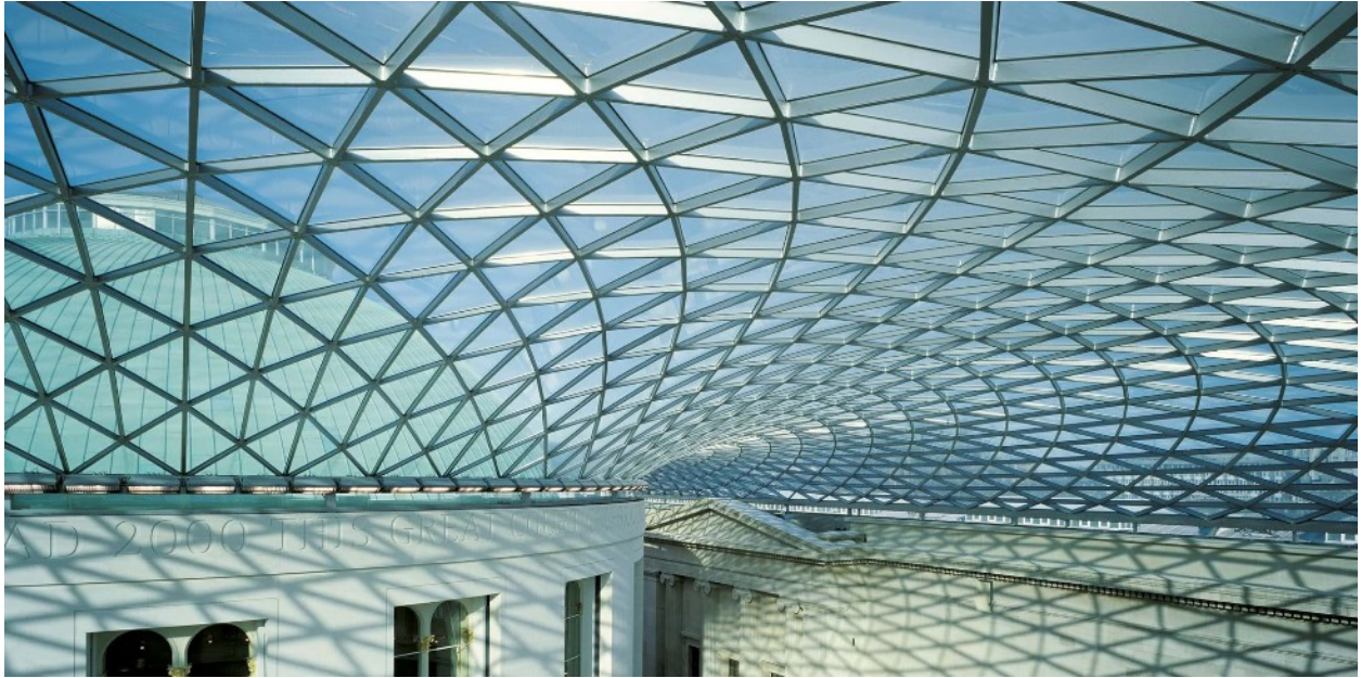
Figure 8. Photo of triangular roof over Great Court in British Museum, London. Designed by Foster+Partners. Image source: fosterandpartners.com
