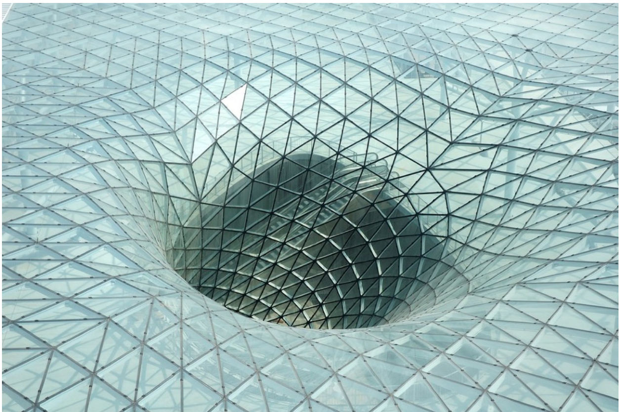
Figure 9. Close-up of roof of New Milan Trade Fair by Massimiliano and Doriana Fuksas. The transition from quads on the planar parts to triangles on the curved parts is evident. Image source: Archive Fuksas.
