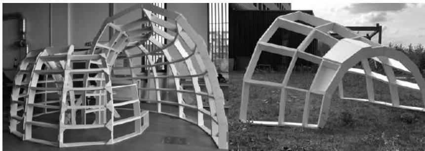
Figure 5: Left: The pavilion with torsion-free nodes. Right: Planar quadrangles used as bracing. (Mesnil, 2017)
